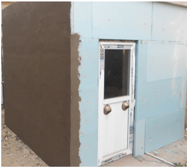
Fig. 3. The picture of the test room.
